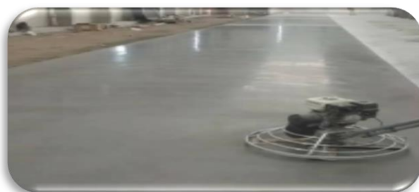
Fig 1: factory floor achieved by Novo Corundum
